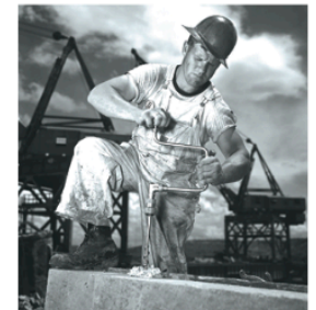
Carpenter working on Douglas Dam in East Tennessee
