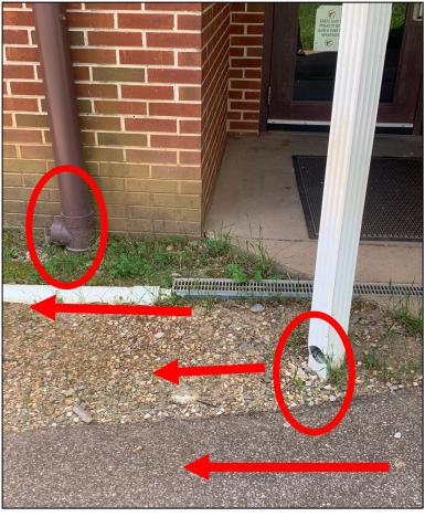
**K-2 Exit to Playground from School Building:** Ss line up here to go inside; drainage of mud onto sidewalk is an issue; note the drain pipes that flow into the area and water from hill
