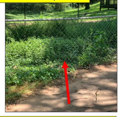
**K-2 Backside of Playground at Corner of Track:** water flows down from grassy hill and building; water also flows down the sides of the track (no drain grate) to the reservoir at fence.
