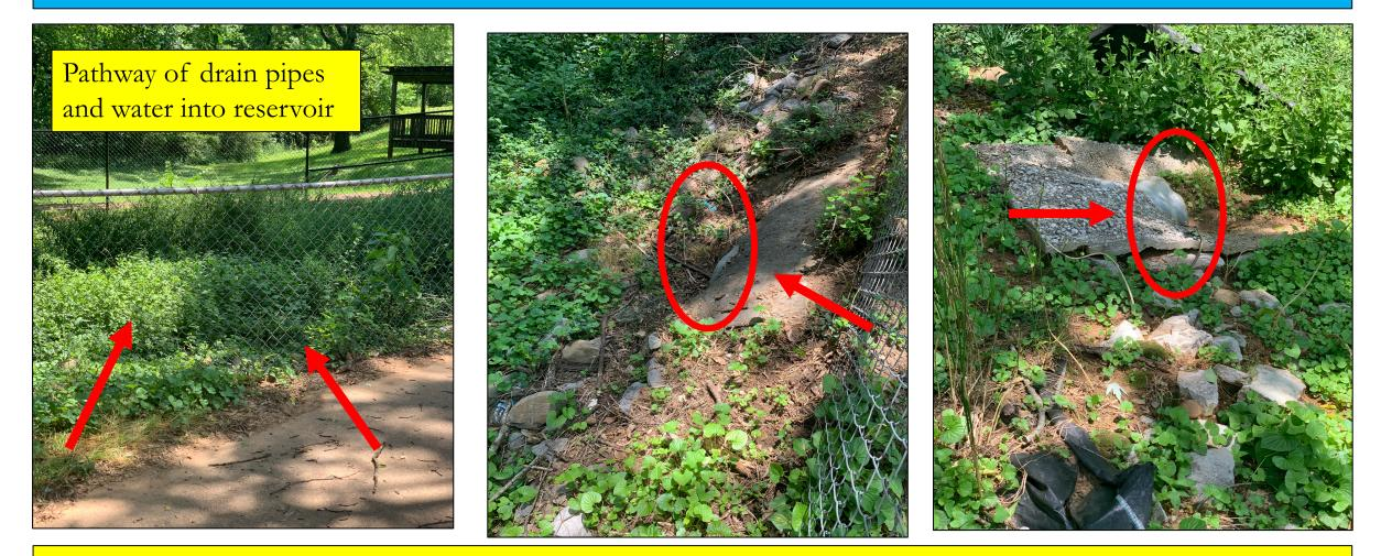
**K-2 Backside of Playground at Corner of Track:** reservoir has two pipes showing the end of the French drain system; would tie all drainage pipes to this system
