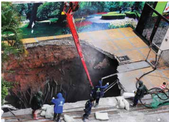
A large sinkhole appeared suddenly in a street of Shenzhen, China. A security guard fell into it and died.
