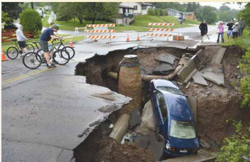
A sinkhole opened in Duluth, Minn., on June 20, 2011. Steady torrential downpours caused residents to evacuate their homes and this car to fall into the sinkhole.
